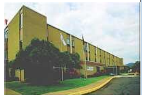
Summers County ARH Hospital
